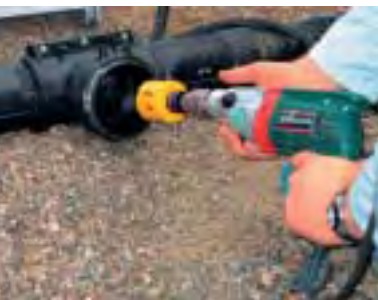
Calyx drill for pressureless tapping – efficient pipe laying
