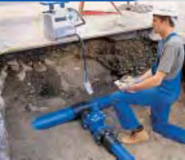
Efficient and safe jointing with MSA electrofusion control units
